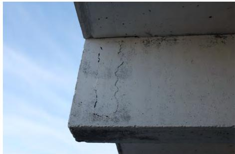
(f) Damage category 3, console bottom. Large cracks, will lead to broken off concrete.
