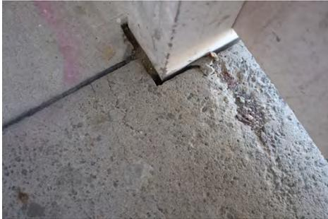
(c) Damage category 2, plate. Spalling of concrete, loose concrete surface, small cracks.
