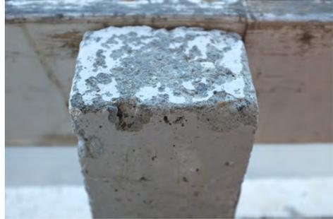
(b) Damage category 1, console top. Slightly uneven top surface, no signs of cracks.
