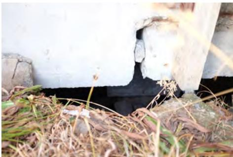
**Figure 3.23:** View of bearing pile under building.
