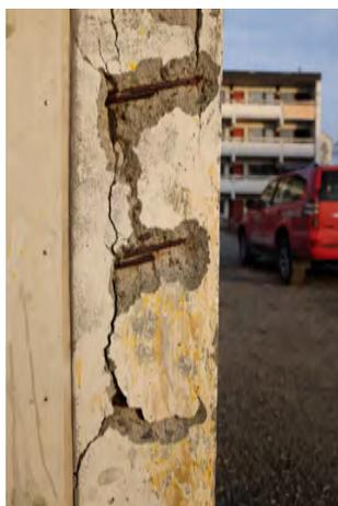
**Figure 3.19:** Damages on column.
