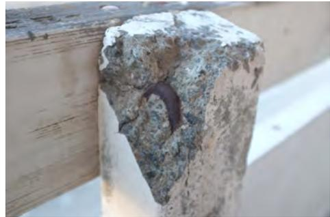
**Figure 3.33:** Aggregates in concrete, block 10.
