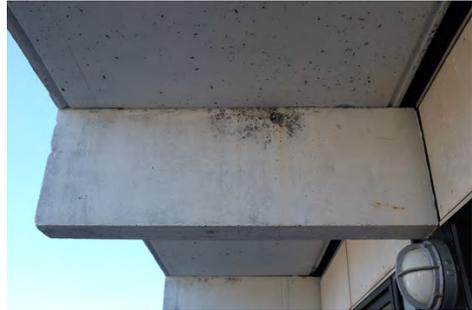
(d) Damage category 2, console bottom. Uneven concrete surface patch, signs of cracks.
