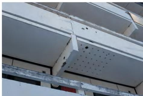
**Figure 3.31:** Holes in the elements due to previous drill core testing.
