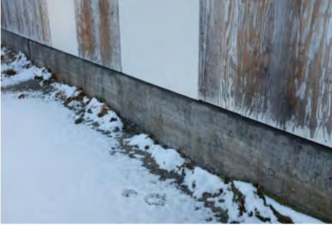
**Figure 3.27:** In-situ cast foundation of block 7.
