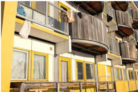
**Figure 2.4:** Rounded steel balconies.
