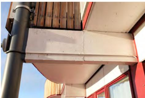
**Figure 3.34:** Renovated block, elongation of console.
