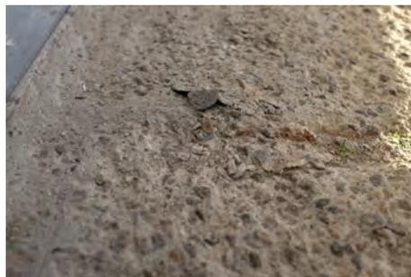
**Figure 3.18:** Uneven concrete surface.
