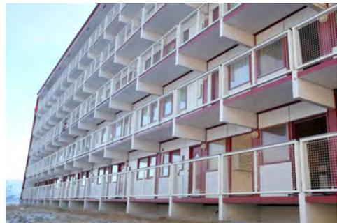
**Figure 3.35:** Renovated block, facade with long consoles.
