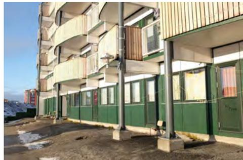
**Figure 2.5:** Asymmetrical concrete balconies.
