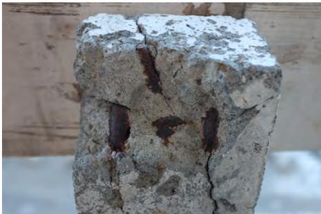
(e) Damage category 3, console top. Large cracks, broken off concrete, visible reinforcement.
