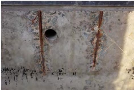
**Figure 3.21:** Corroded reinforcement along the foundation.
