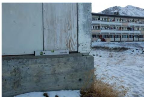
**Figure 3.25:** Placement of spirit level on the foundation.
